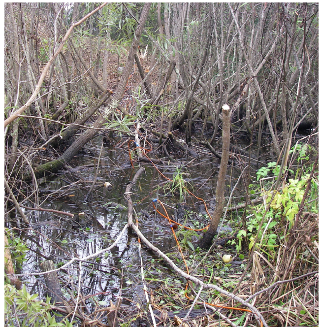
Proper Clearing: Straight line clearing (root and larger tree removal not required)
