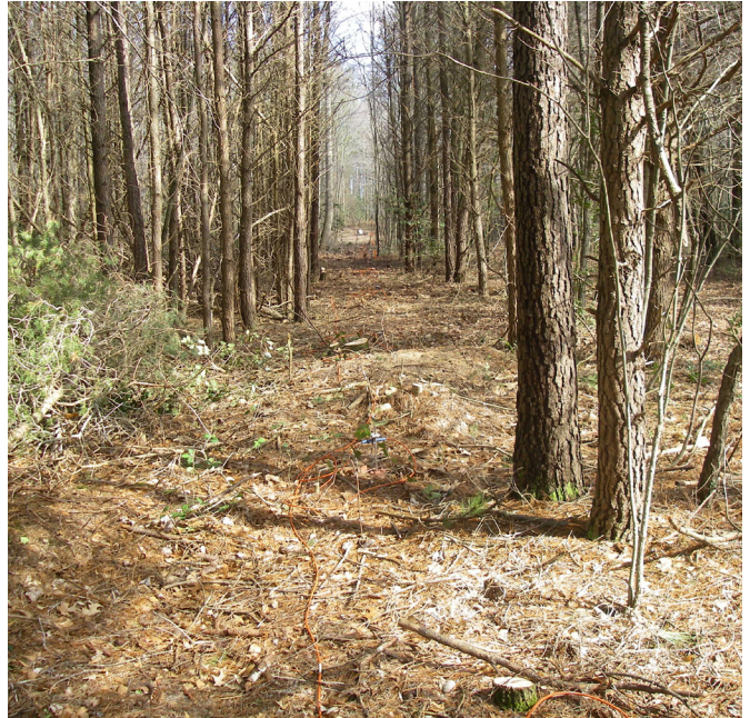
Proper Clearing: Straight line clearing (root and larger tree removal not required)
