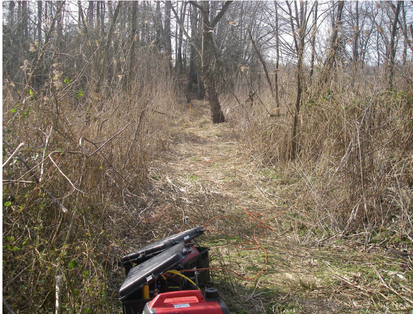
Proper Clearing: Straight line clearing (root and larger tree removal not required)
