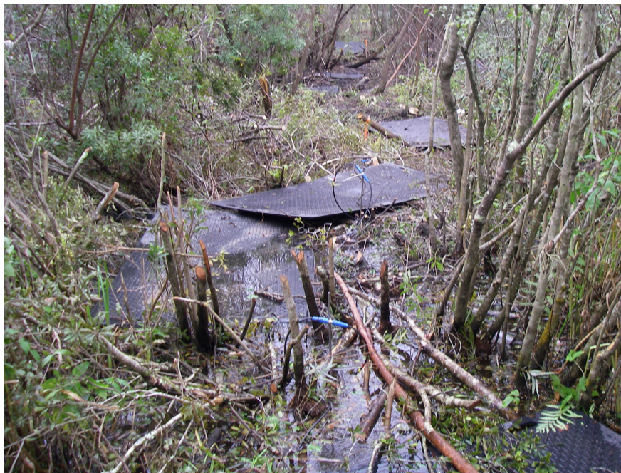
Unacceptable Clearing: Trip Hazards, Not in a Straight Line
