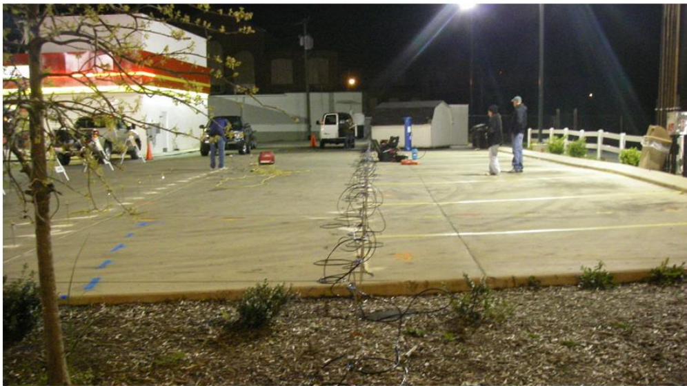
Figure 3: View of ERI line JAC-07 looking north at the former Boone Dry Cleaning facility in Jackson, TN. Data were collected at night to minimize disruptions to businesses currently located on the site.
