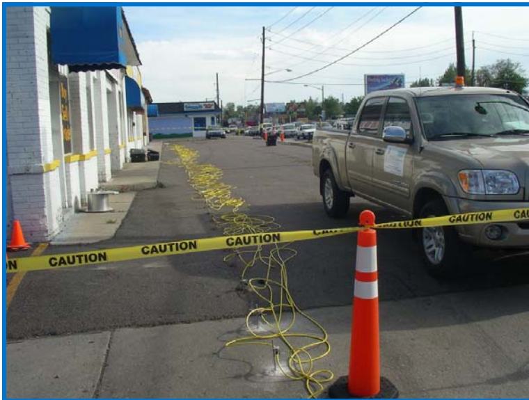
Photo of GeoTrax Survey™ transect with electrode stakes in pre-drilled 1/2-inch diameter holes through asphalt pavement.
