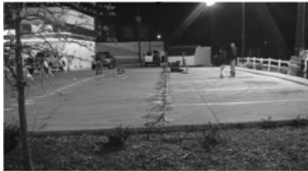
Exhibit 2. Photograph of the deployment of ERI lines at former dry cleaners in Jackson, Tennessee
